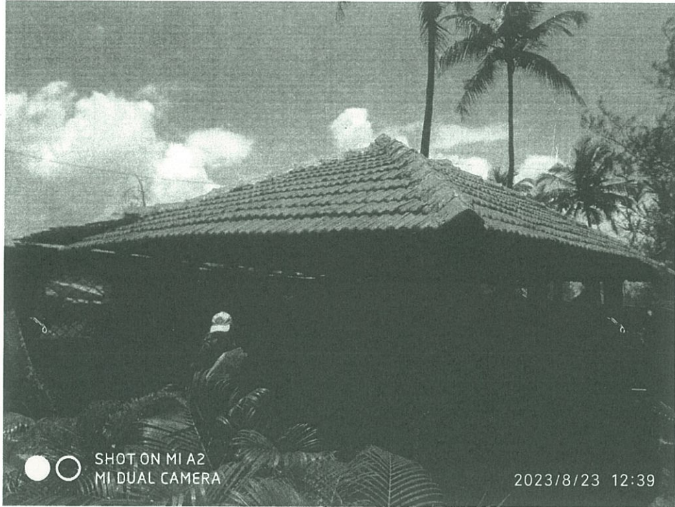
(c) SHED WITH MANGALORE TILE ROOFING
