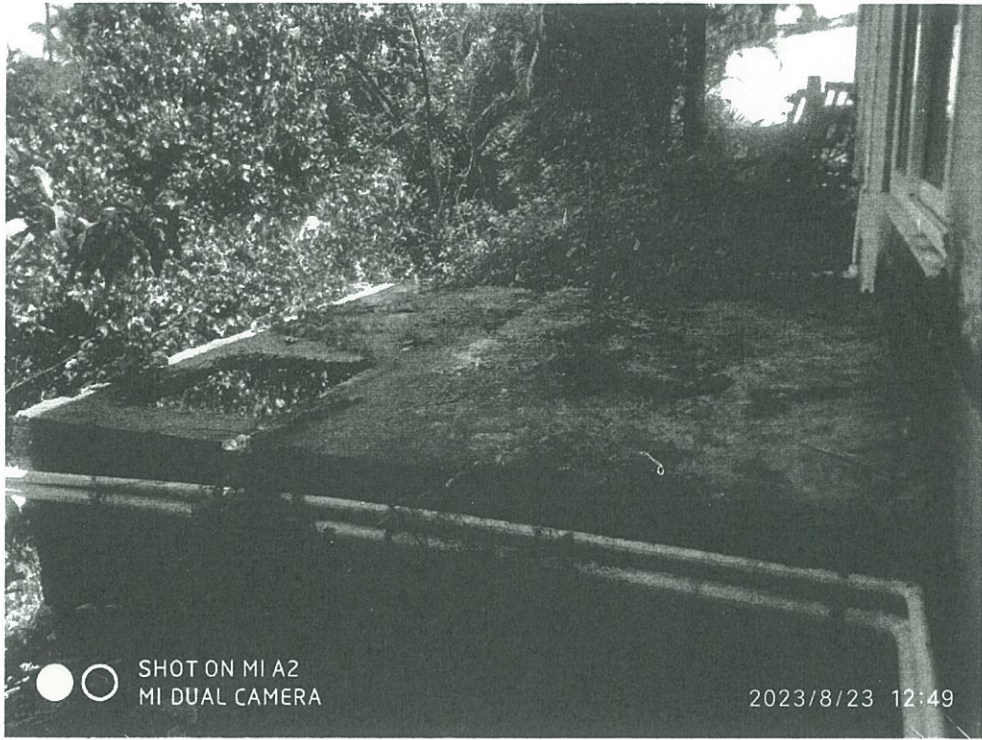
TANK 2 ATTACHED NORTH-EAST SIDE OF STRUCTURE 'C'
